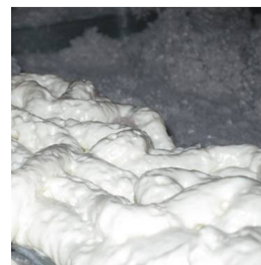
Combination of air sealing and blown-in insulation
