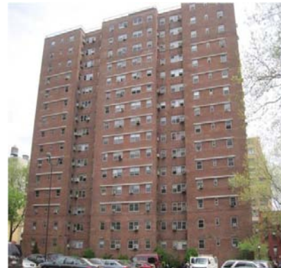
3. Post-War two-pipe steam
