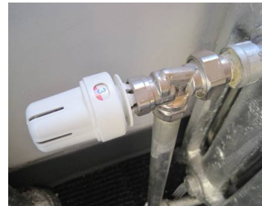
Thermostatic Radiator Valve (TRV)
