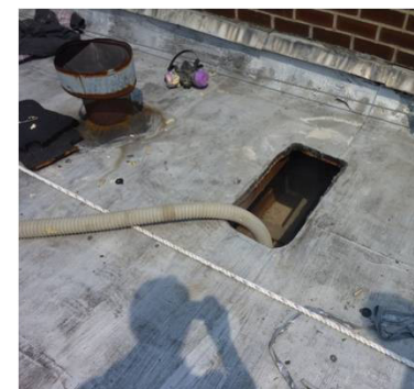
Cavity between roof deck and top floor ceiling
